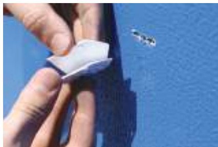
2 Take two Styrowedge halves and join the smooth sides together.
