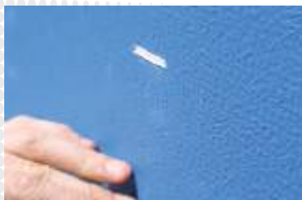
4 Ensure the Styrowedge is flush with the finish of the wall.
