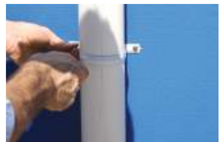
6 Complete for remaining fastenings. NB. Ensure all penetrations are sealed.
