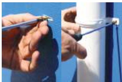
5 Place the downpipe and clip in position on the wall. Insert an 8-12 gauge screw into the Styrowedge and tighten into place.
