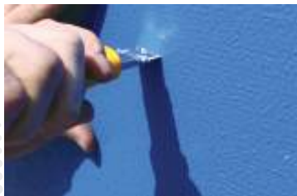
1 Using a sharp blade, cut a 30mm slot, 50mm deep into the wall.
