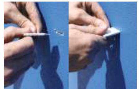
3 Insert the Styrowedge into the slot in the wall.
